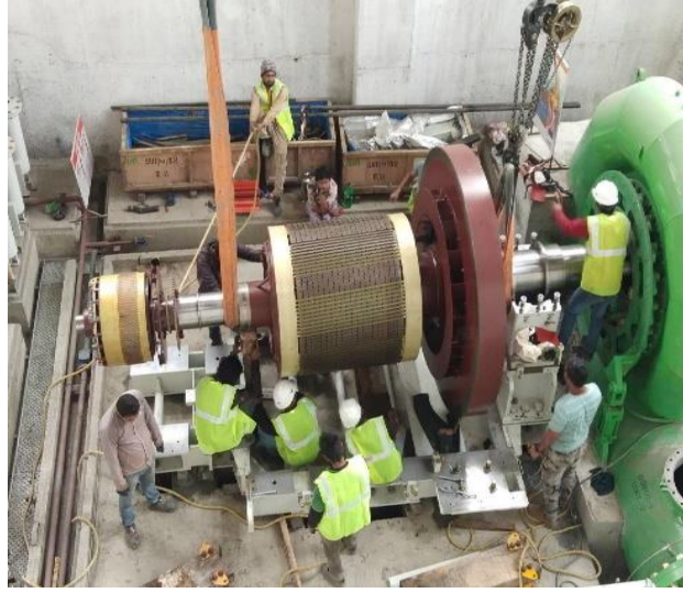
Rotor Positioning inside Powerhouse
