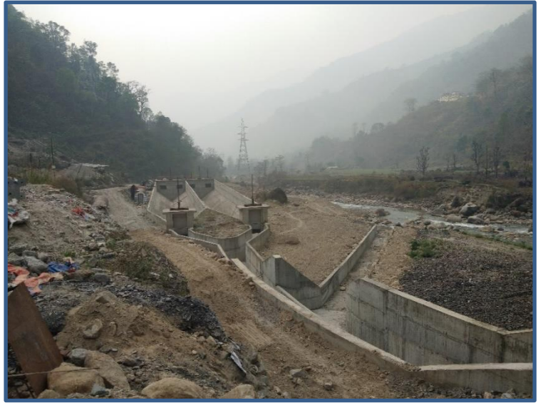
Railing and Shades in Headworks.
