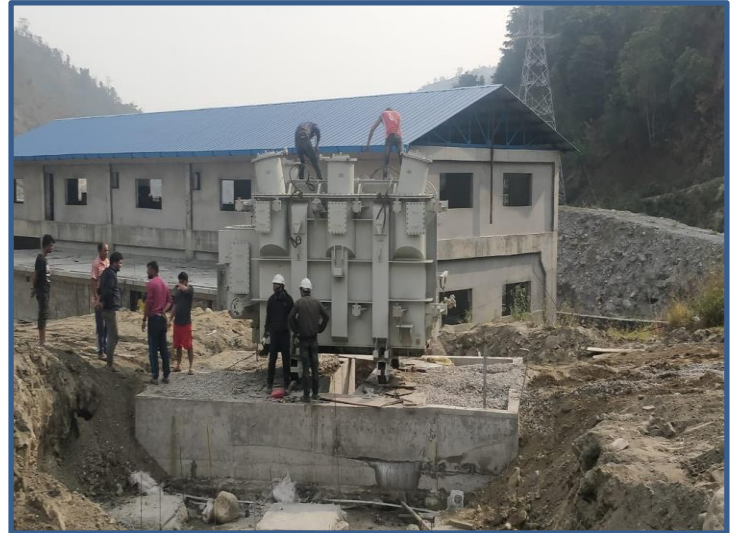
Transformer Unloading
