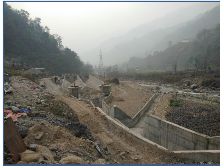
Railling and Shades in Headworks.
