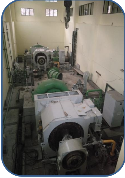
Power House Machine Hall
