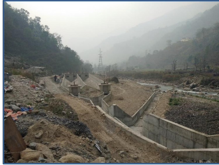
Railling and Shades in Headworks.
