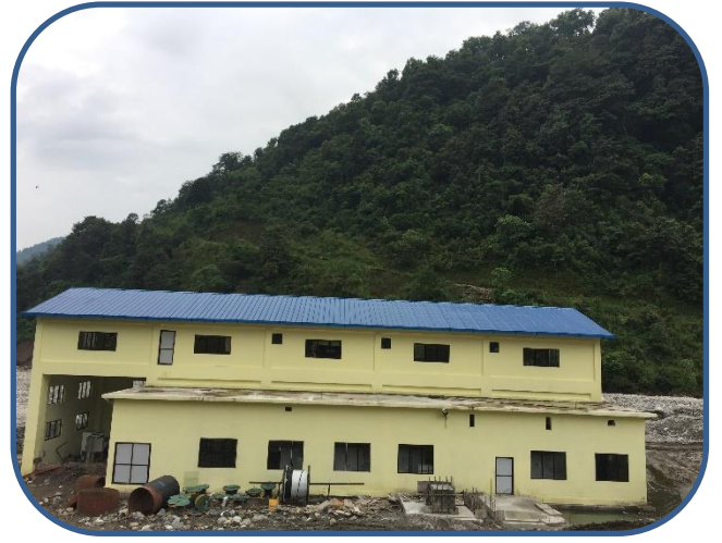
Power House Control Room
