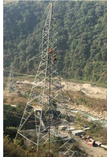
Transmission Line Tower Erection on Progress
