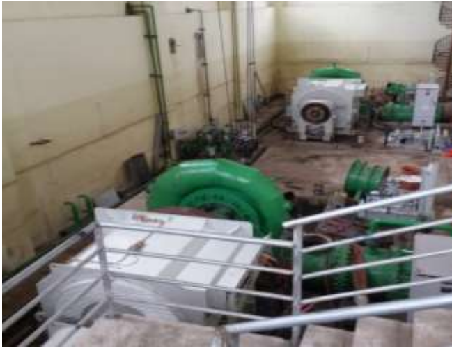
Power House Machine Hall
