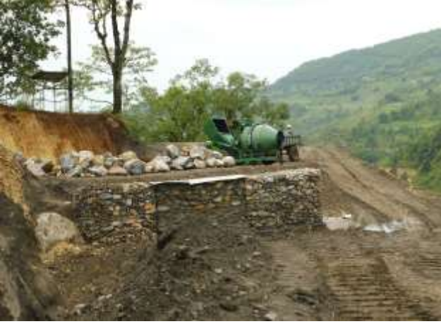
Tunnel Outlet Portal Setup
