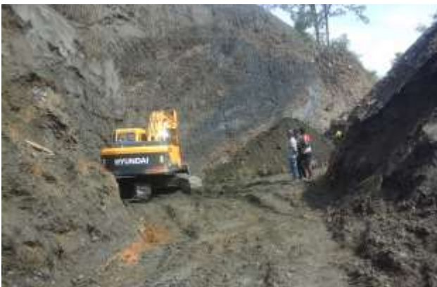
Tunnel Outlet Portal
