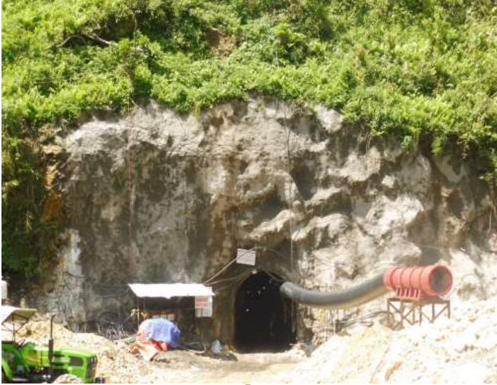
Tunnel Inlet Portal
