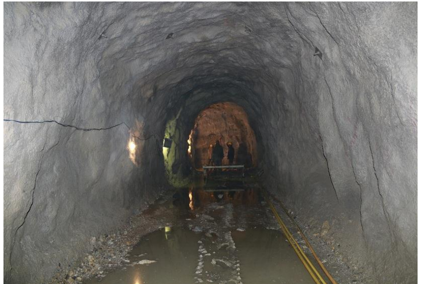
Planning of Drilling works
