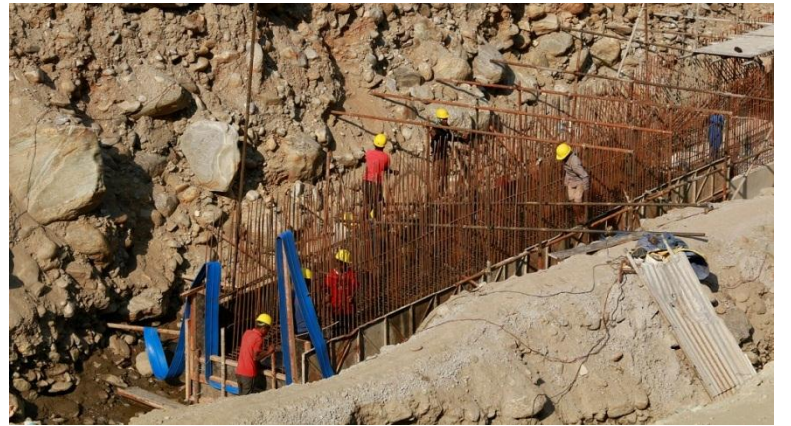
Desander Construction in Progress
