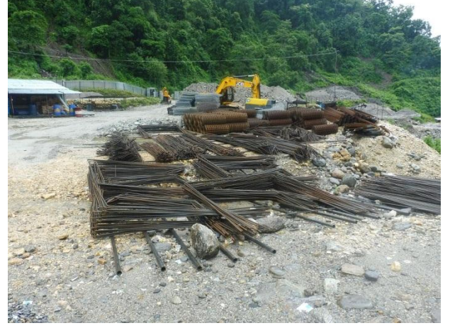
Bar bending works accomplished till date
