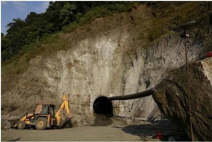
View of Tunnel Outlet Area
