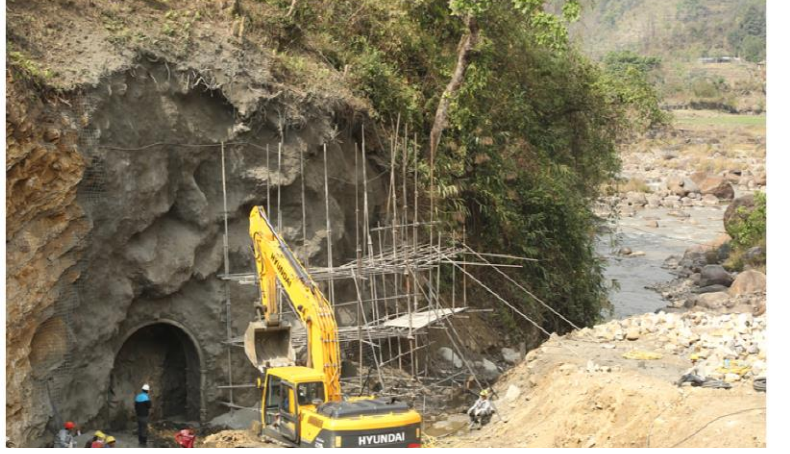
Tunnel Inlet Portal
