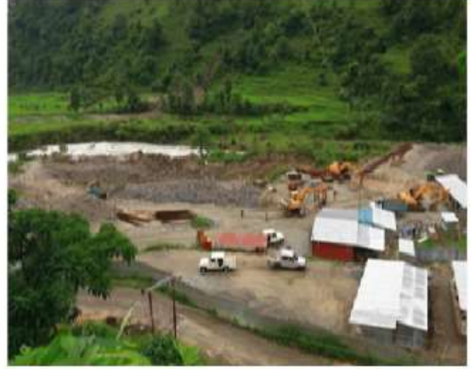
Headwork Site Overview
