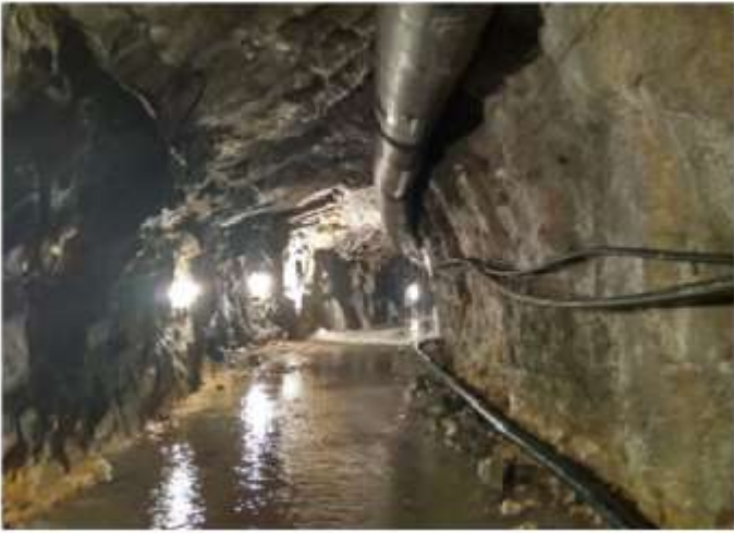
Inlet Headrace Tunnel
