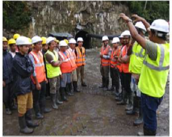
Safety Training at site before work
