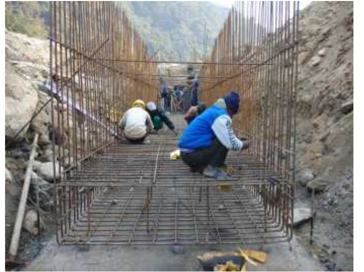
Rebar placing in Desander Purge Canal
