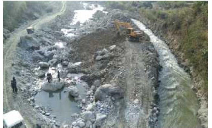
Completion of River Diversion Works
