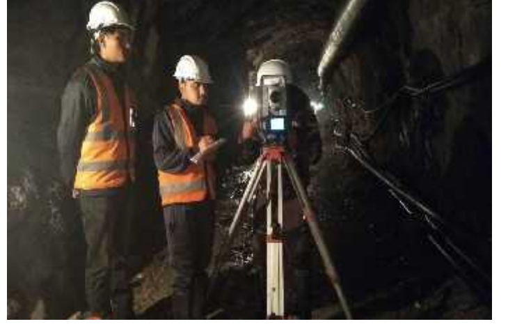
Survey Works Ongoing inside Tunnel
