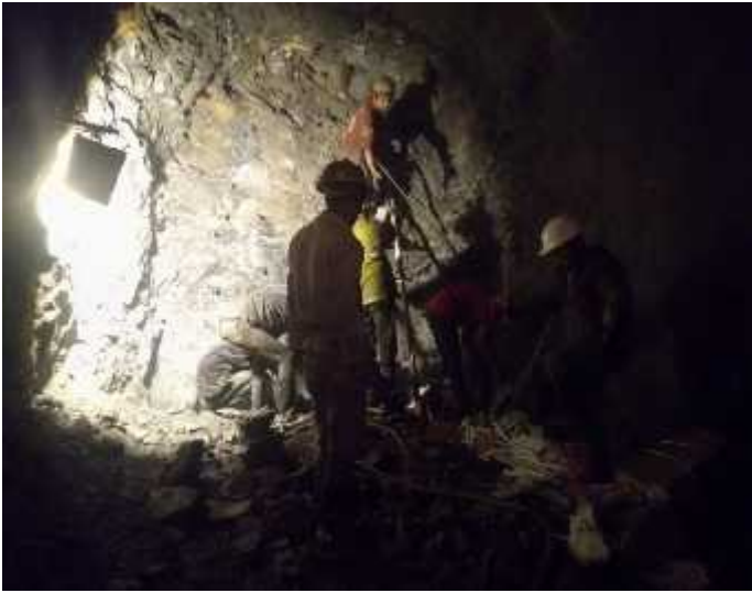
Blasting Preparation - Explosive Packing Works
