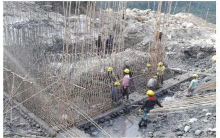
Reinforcement works at Undersluice
