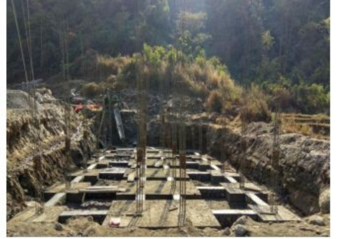
Construction Work of Kirtipur Substation
