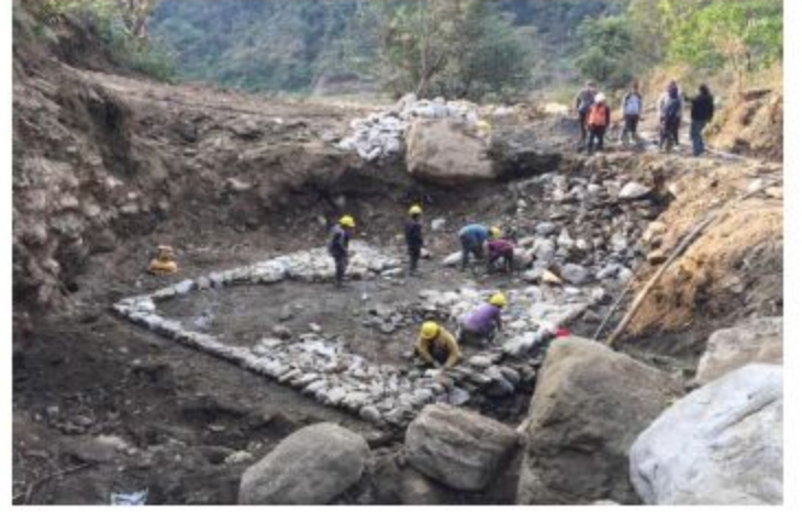
Preparation for foundation works at Penstock Line
